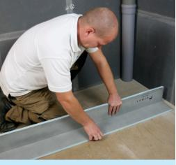
**2** If necessary for extra waterproofing run a bead of Marmox MSP360 Sealant & Adhesive along the fold. Then fold to create a 90° angle.
