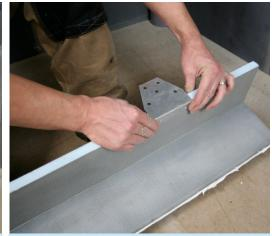
**4** If the Marmox pipe boxing is being used against a solid wall then it is recommended to use Marmox Wall Brackets. Use 2 per side of a 1.25m length.
