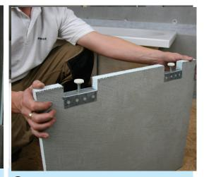
**8** You can seal the edges with Marmox MSP360. The Marmox pipe boxing is now ready to be plastered or tiled.
