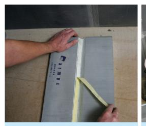
**1** Cut to correct length. They come in 1.25m lengths as standard and cut be stacked on top of each other to create height. Remove the tape.
