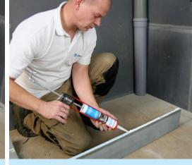
**3** If applying to a stud wall of Marmox Multiboard, run a bead of Marmox MSP360 along the edge of the Marmox pipe boxing.
