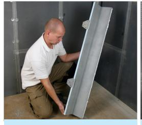
**5** This example shows being fitted in the corner against a stud wall and solid wall. Be sure to mark against the wall and drill out the hole positions.
