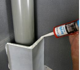
6 Place the Marmox pipe boxing in place and push firmly. Add screw fix-ings. Run a bead of Marmox MSP360 around the top.
