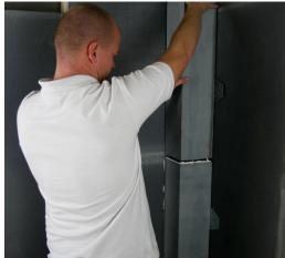
7 Add Marmox MSP360 / Marmox Wall Brackets to the next piece of Marmox pipe boxing and push firmly into place. Add screws.
