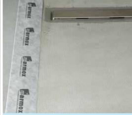
**12** Waterproof all the joints using waterproof tape and waterproof corners then fit the decorative grate, having first inserted the hair trap.
