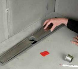
• Using a cement-based flexible tile adhesive, stick the Showerlay to the floor and position the drain tray into position (there is no need to secure this with adhesive).
