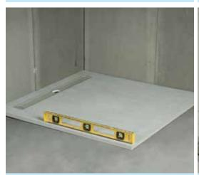
**5** Check that in position, the Showerlay is on a flat surface offering support – especially around the drain.
