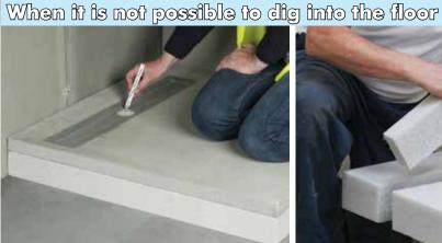
A The 100mm thick plinth will encase the drain and supper the Showerlay.
