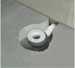
**4** Solvent weld the drain to the BS40mm pipe so it is positioned centrally in the hole.
