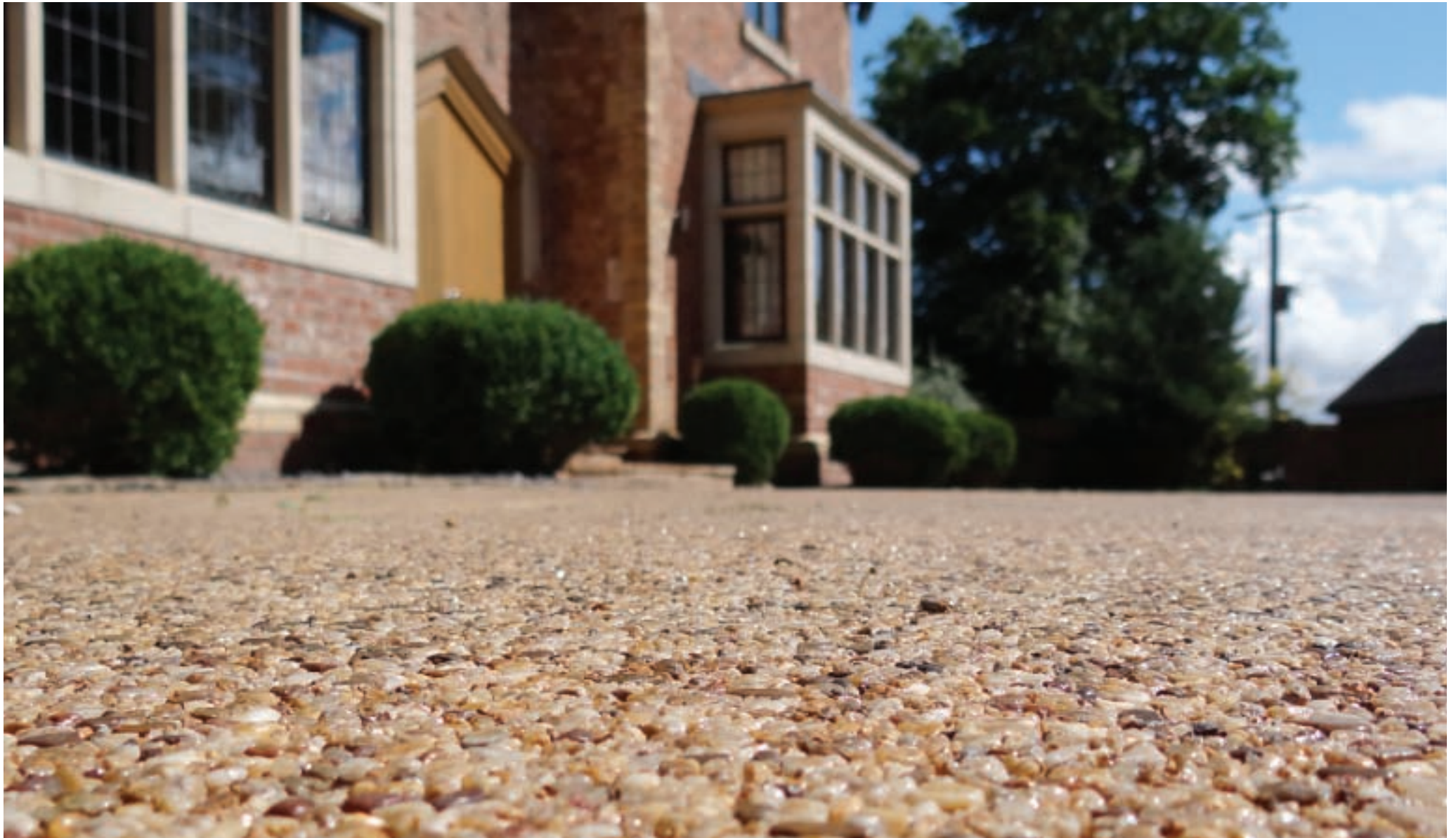
Decra™ Set Fully porous SUDS compliant system, allowing water and air circulation to improve areas prone to standing water.
