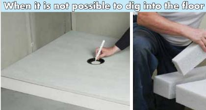
A The 100mm thick plinth will encase the drain and support the Showerlay.
