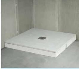
**D** Connect the gully to the drain pipe, fix the Showerlay to the plinth using a flexible adhesive and continue from step 5 above.
