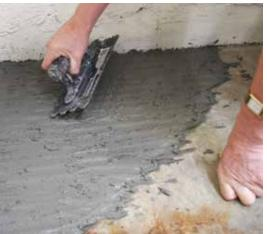
**C** Fix down the Plinth to the floor using a full bed of flexible cement based tile adhesive. Use the adhesive to help level any uneven floors.
