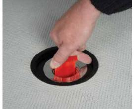
7 Screw the flange ring through the Showerlay into the drain below. Hand-tighten using the red "key". No sealants should be used.
