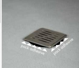
Check that the height of grate in the silver frame will be level with the tiles when fixed with adhesive. To secure and stabilise the drain frame, pack some tile adhesive underneath.
