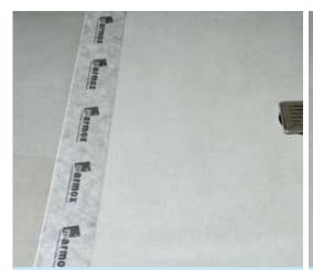
**9** Tape joints using Marmox Self-Adhesive Waterproof Tape.
