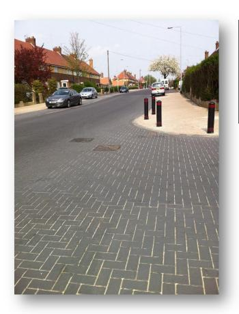
HMS Decra®Print Imprinted surfacing is a hot applied resin based compound. It is a modern alternative to blocks, slabs, and cobbles.
