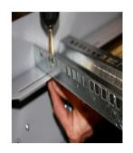
Attach vertical infill panels to the front right and left profiles only. NB these are only used on 800mm wide cabinets.
