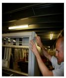
Insert roofing bolt through the top cover and then through aluminum spacer and screw into captive fixing in top of cabinet.
