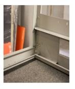
Fix with M6 x 12mm screws in each corner.
