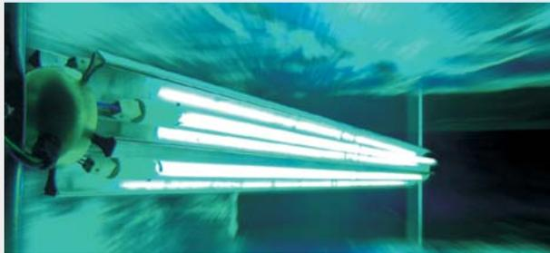
Installing parallel to the air-stream increases dwell time (contact time) with air
