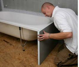
3 Measure and mark the smallest panel against the end of the bath. Be sure to leave a 30mm gap on the outer edge for the side panel to sit in front of.
