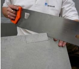
**6** Cut out the marked section using a saw or knife.
