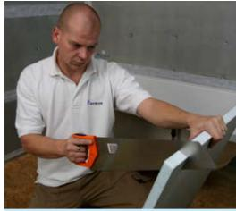
**4** Cut the panel to size using a saw.
