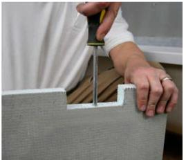
**7** Drive a screwdriver into the panel in the centre of the cut out section to allow the bolt to sit inside the foam.
