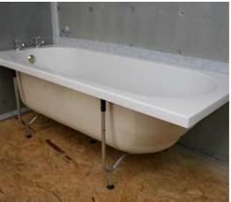
**2** Position the bath and make sure you have enough room to allow a 30mm panel to fit under both sides. Move legs over if necessary.
